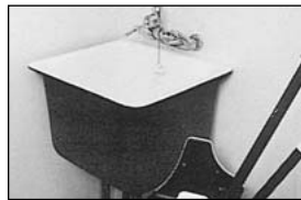
SERVICE SINKS - Maintenance and janitorial clean-up areas.
